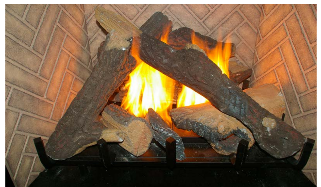
Figure 18m. Completed Log Set Installation.
