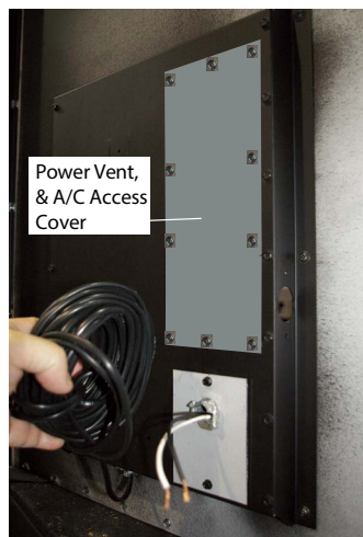
Figure 12a. Remove Exterior Access Cover.
