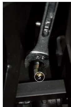
Figure 20d. (Loosening Gas fitting on burner).
