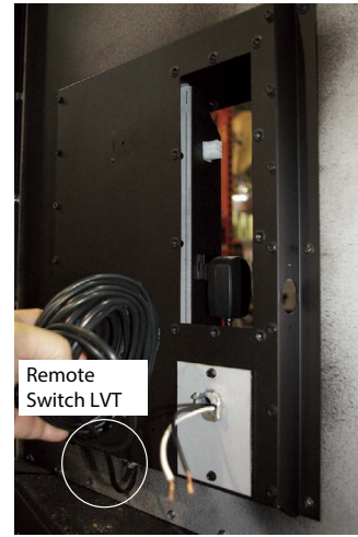
Figure 12f. Installing the Remote LVT Switch.
